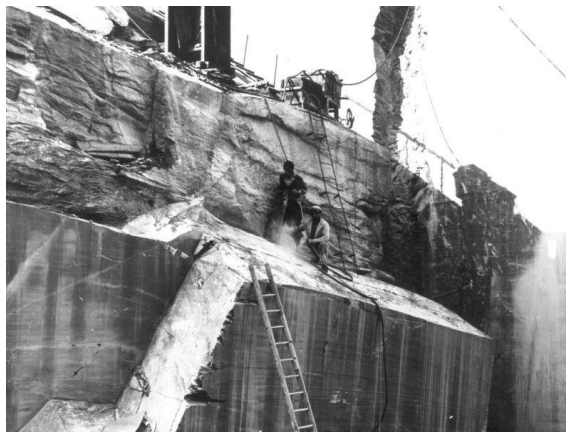
picture 1 Mine hole preparation in a serpentine quarry.
