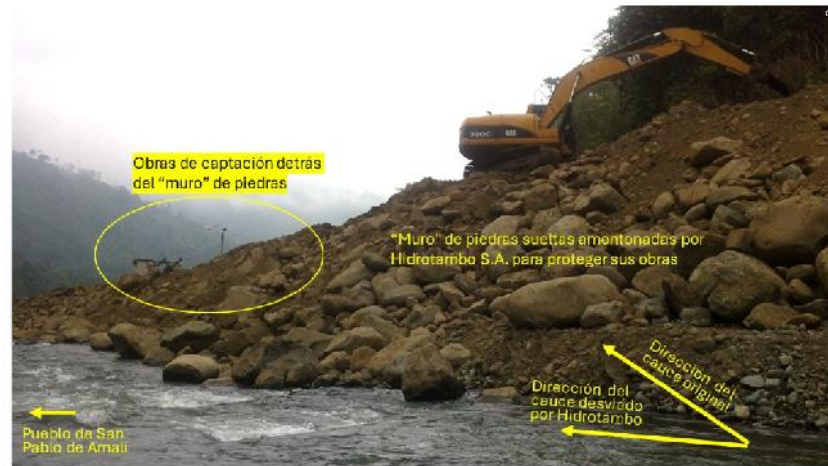
Figure 3.4 The Hidrotambo wall to protect its infrastructure. Source: Rachel Conrad, 2015.
